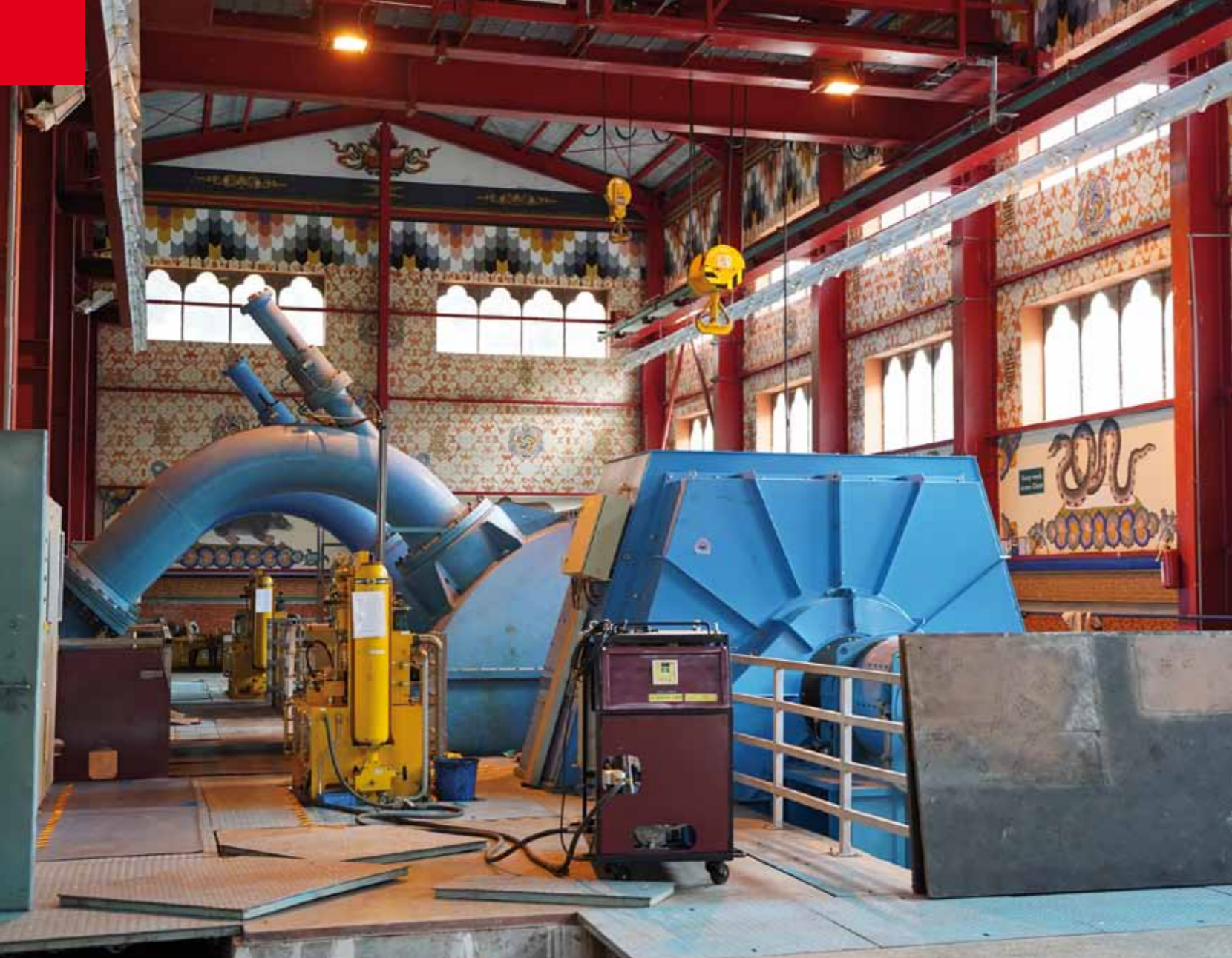
Turbine at Basochu hydropower station
